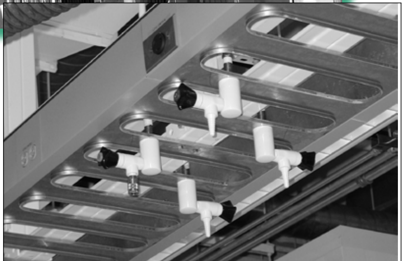
Series 6 Trough Cable Tray Typical Installations
