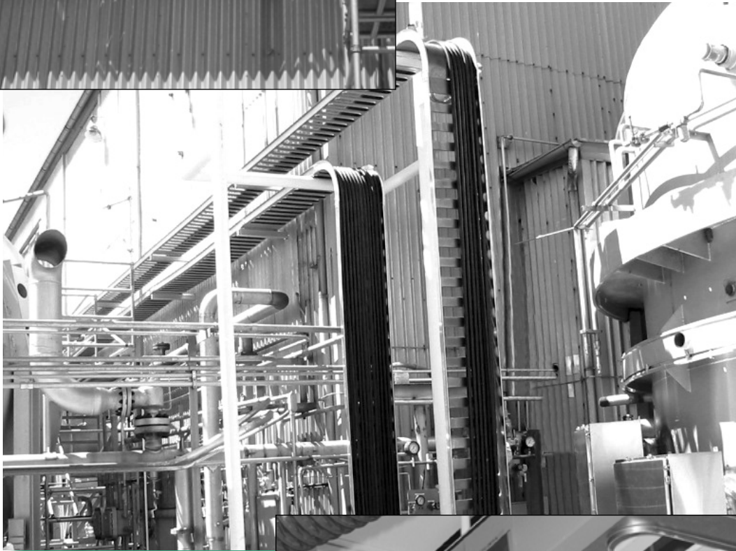
Series 6 Trough Cable Tray Typical Installations
